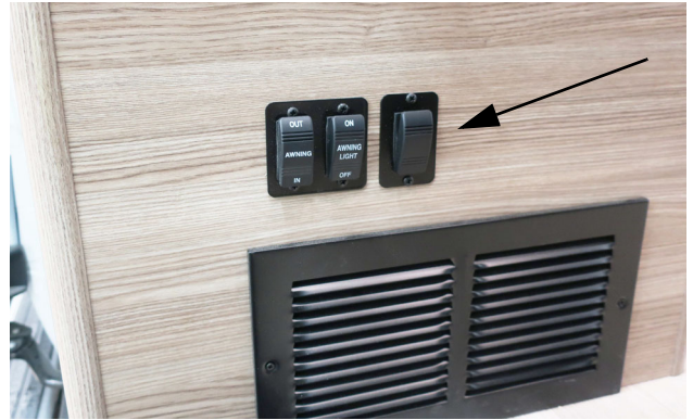
Accent LED Running Board Light Switch (Located near sliding entrance door) -Typical View
