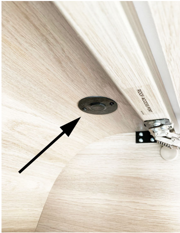
Roof Access Port -Typical View
